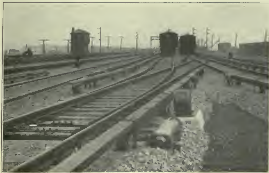
FIG. 507. THIRD RAIL CONTACT SYSTEMS. Construction at Switches, 600-Volt Over Running Third Rail Installation, Pennsylvania Railroad, New York City.
